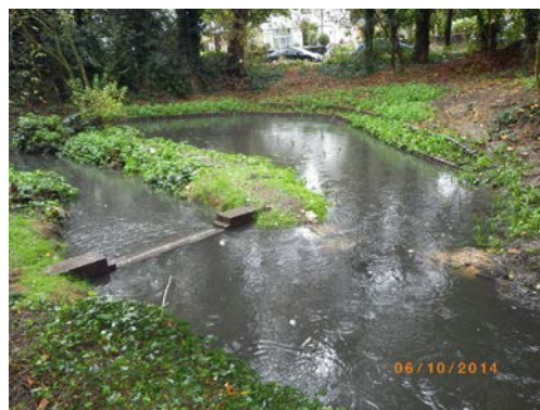
Figure 3.6 Bioretention SuDS cells at Glenbrook, Lonsdale Drive
