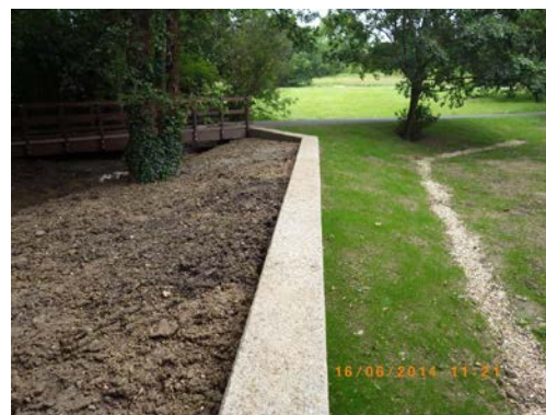
Figure 3.4 Flood defence wall at Grovelands Park
