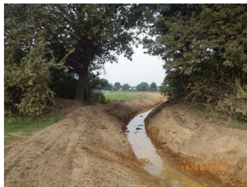
Figure 3.2 River restoration works in progress at Firs Farm Playing Fields
